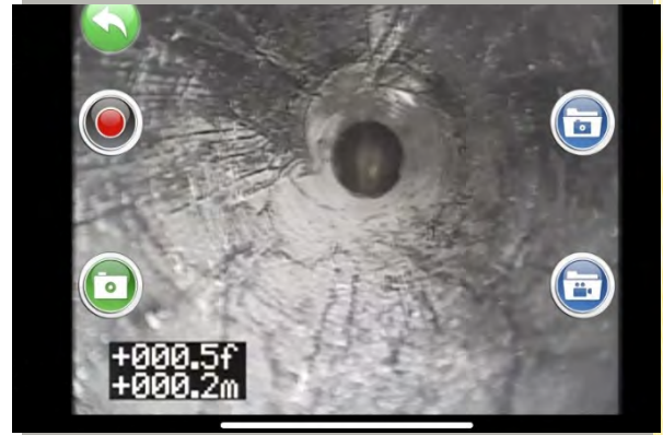
Actual screen shot taken on an iPad from a mini camera in a 3" pipe.
